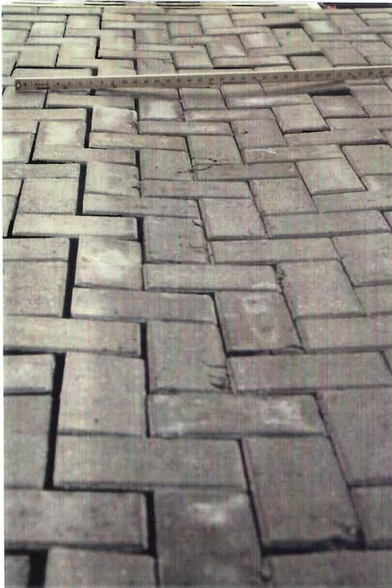
Renewed Rectangular Paving Stone Section (90° Herringbone Pattern), again showing severe deformation, Summer 94 Please note that the UNI-ANCHORLOCK® Section is the same as in the earlier test!
